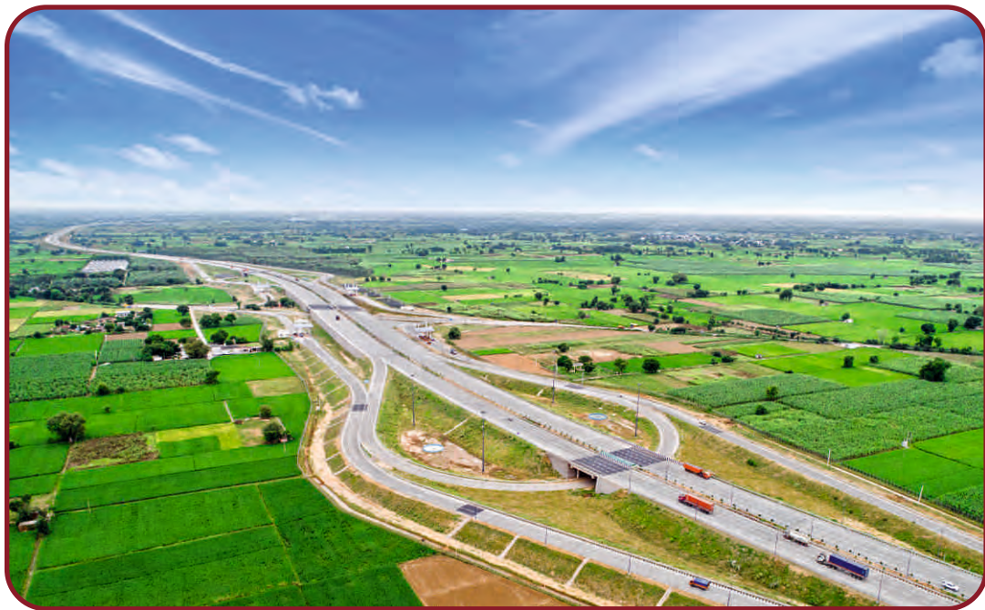
Eastern Peripheral Expressway
